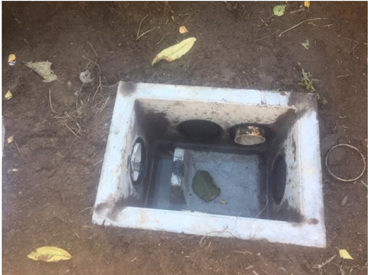
New d-box back filled
